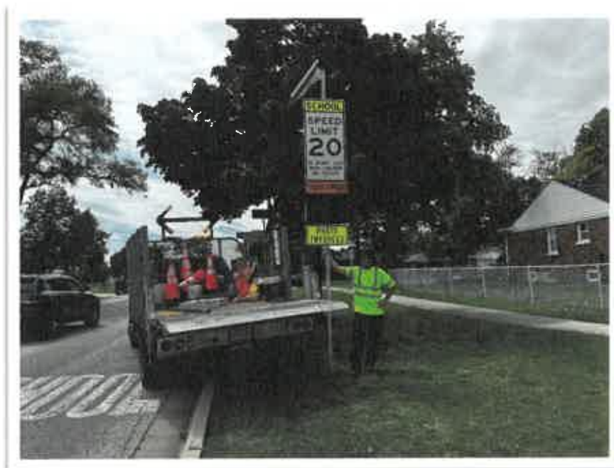
The sign crew installs a "School Zone" sign on Fullerton Ave.
